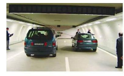
For urban tunnels, international practice reveals design solutions of great value. Such an example is the A86 Duplex Tunnel part of Paris Super-Peripherique, completed in January 2011. It is an innovative 10km tunnel, with a diameter of 10.4 m, exclusively for light vehicles and features two decks each with two traffic lanes and an emergency one. Each level is independent of the other.
