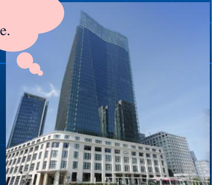
JP TOWER Hall & Conference
