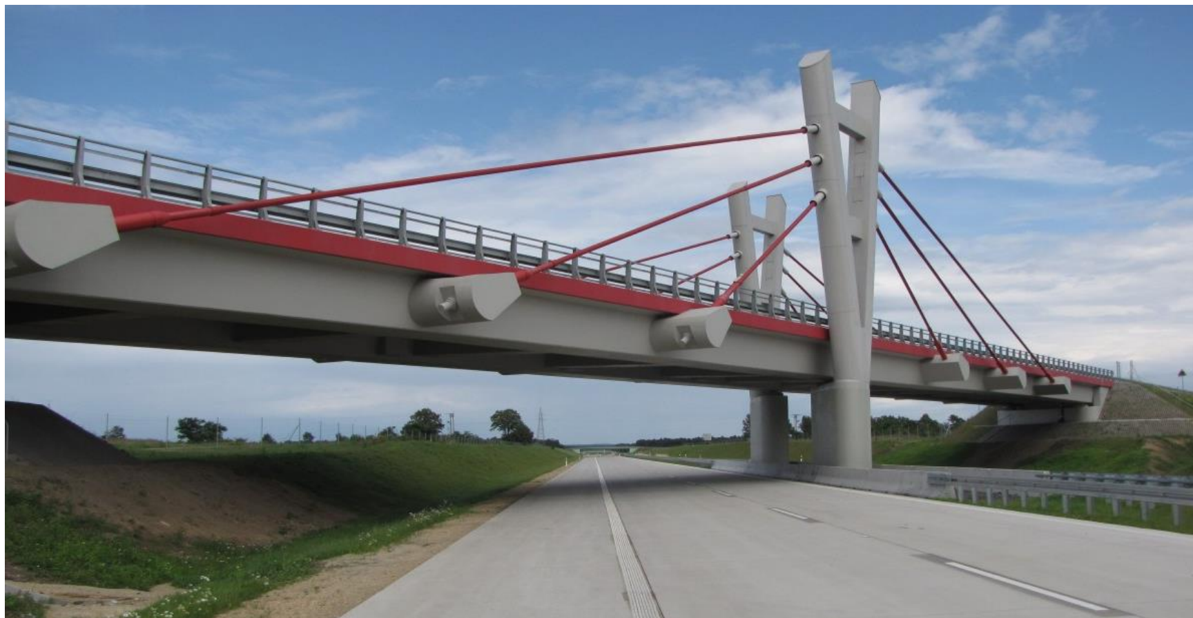
View of completed viaduct
