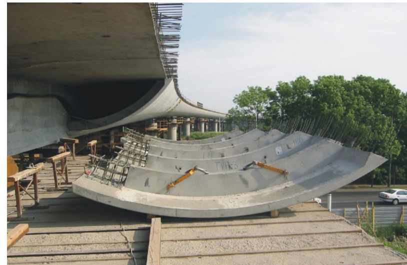
View of the Gądowska flyover and view of side precast elements
