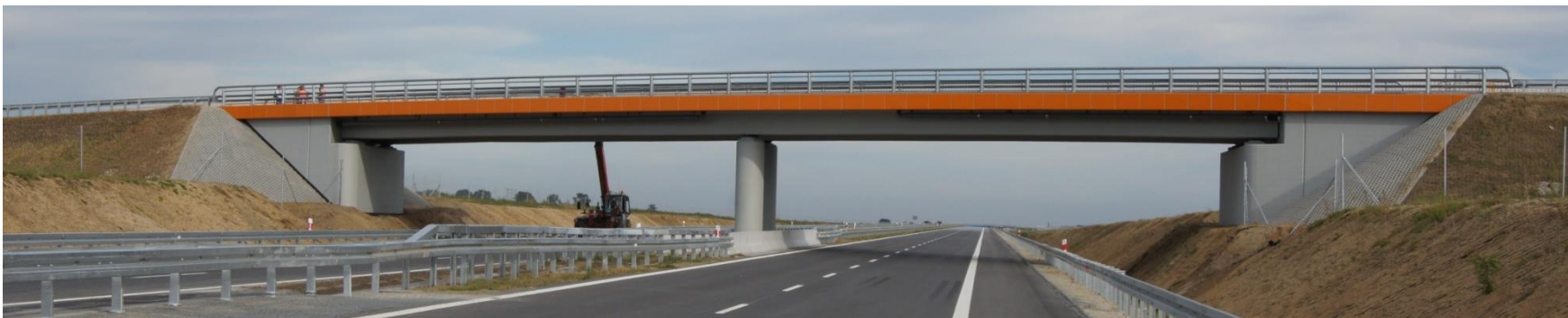
Beam viaducts over the S8 expressway
