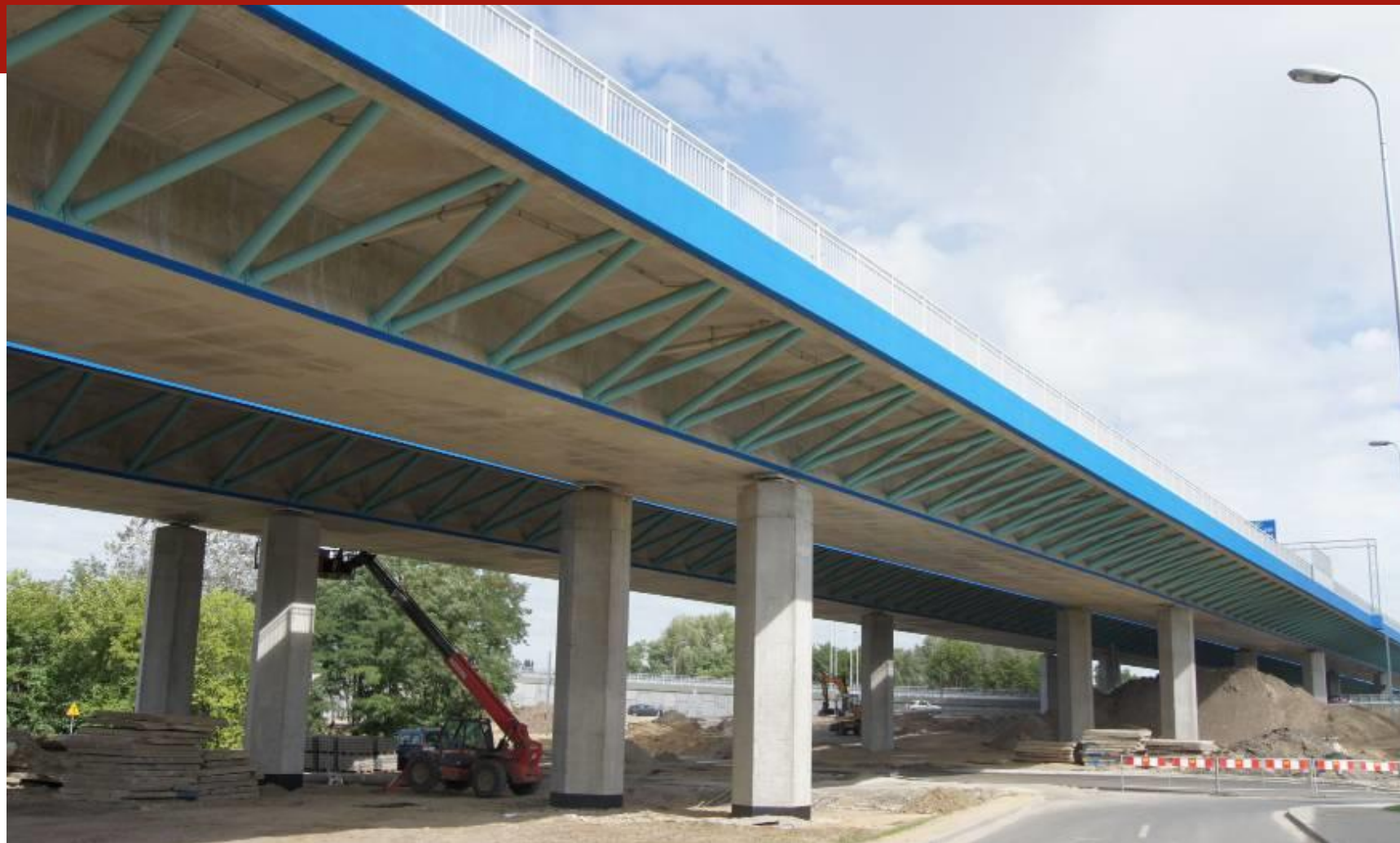
Completed WA-19 flyover
