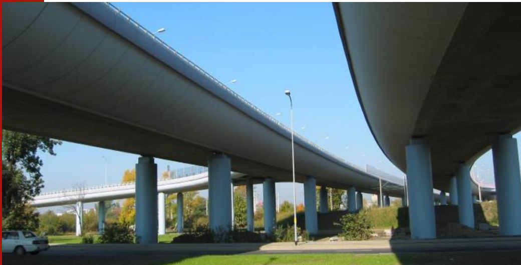
View of the Gądowska flyover and view of side precast elements
