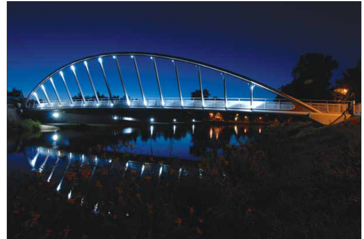
Bridge over the Vltava
