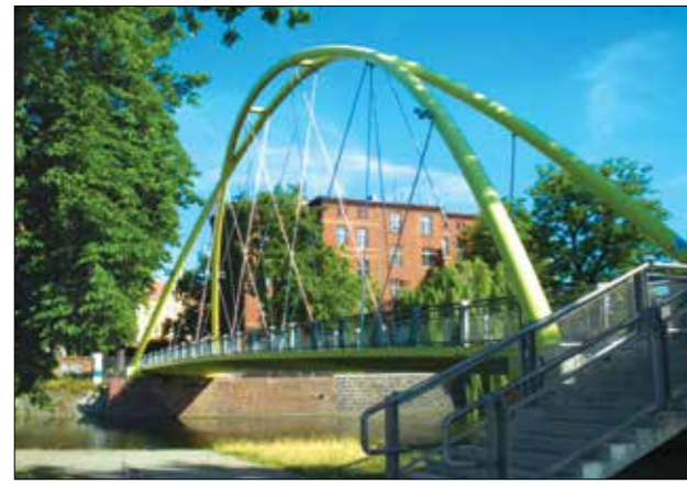
Malt Island Footbridge over the river Odra
