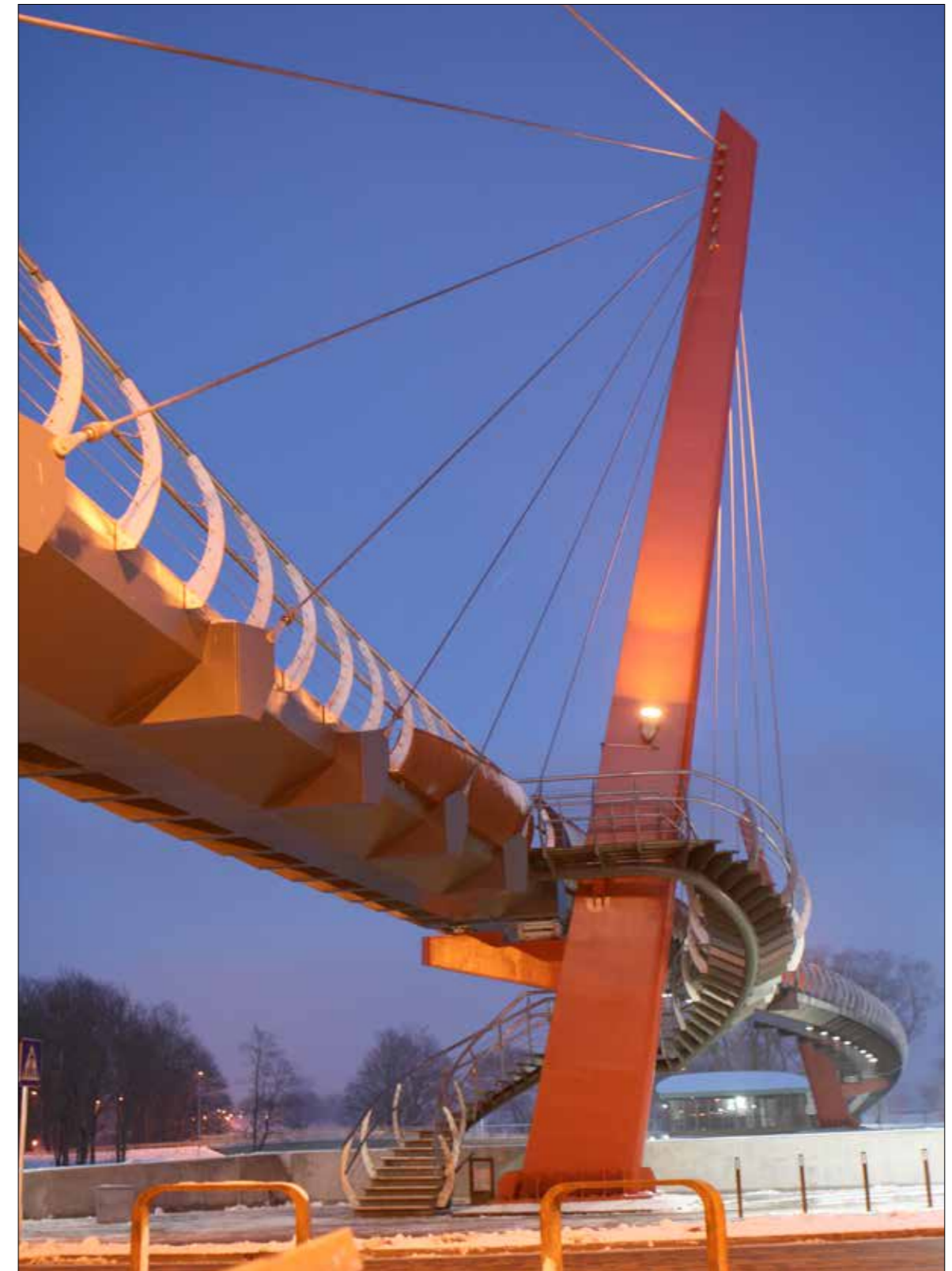
Mitava footbridge over the river Driksa
